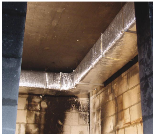
Fig. 12 - Fitting of the duct made of galvanised steel insulated with fibre glass
