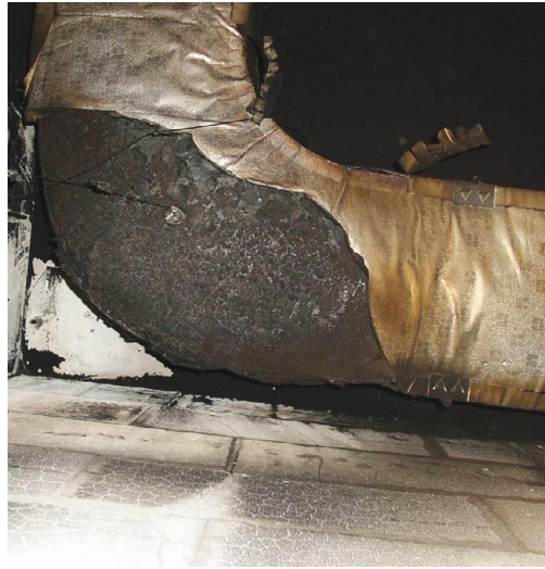
Fig. 16 - The P3ductal duct shows the effects of the fire only in the area hit directly by the flames
