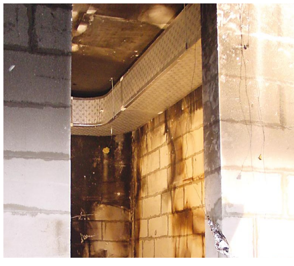
Fig. 8 - Layout of the room used for the room corner test
