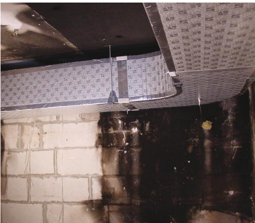
Fig. 11 - Fitting of the preinsulated aluminium P3ductal duct
